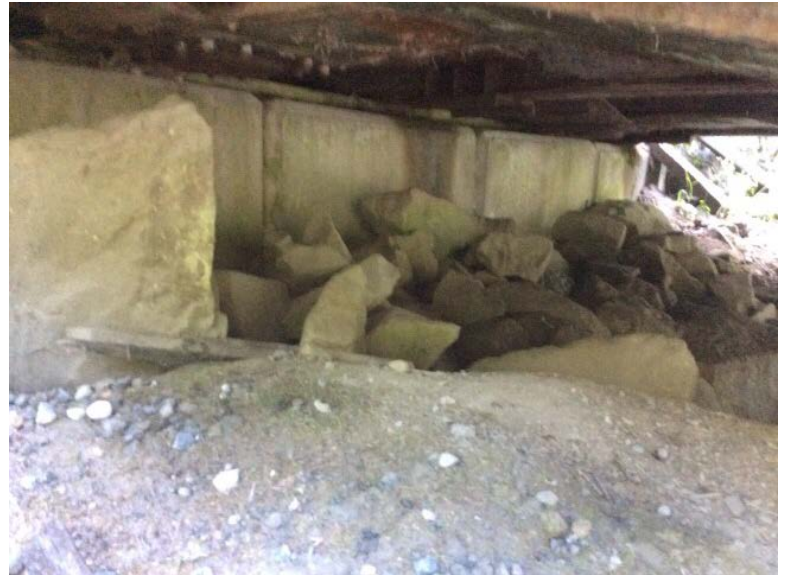
Left Bank Abutment when facing downstream
