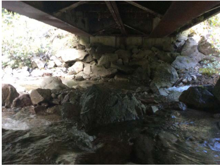
Right Bank Abutment when facing downstream
